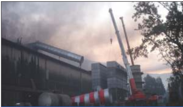
Erection of Secondary FES for 50 Ton EAF handling 600000 MCH volume
