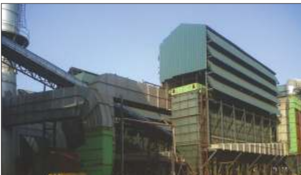
Installation and GCPs on 4 x 9 MVA furnaces handling 5,20,000 MCH volume
