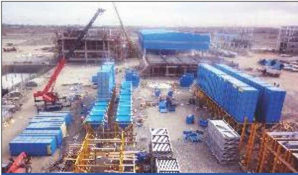
Erection work of GCP in progress at OMAN
