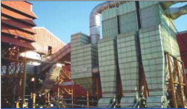
Gas Cleaning Plant on 25T EAF and 25T LRF- Zambia
