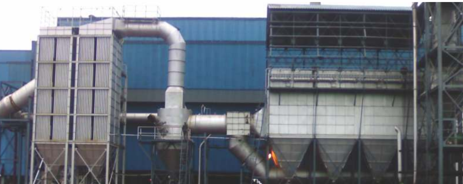
Gas Cleaning Plant for 50T EAF & LRF
