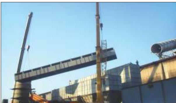
Erection of Plenum
