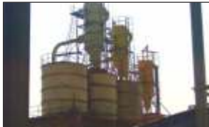
Baghouse on pneumatic conveying and drying application
