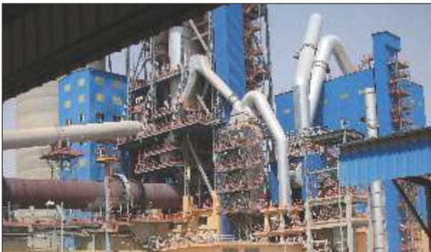
Cement Mill section where revamped baghouses installed
