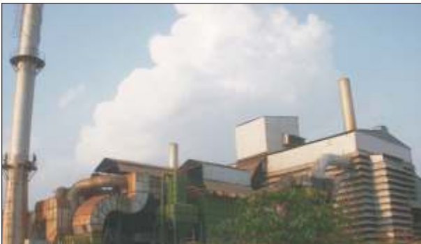
Installation of GCP on 2 x 27 MVA furnace handling 540000 MCH volume
