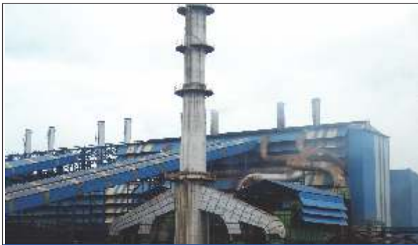
Installation of GCPs on 4 x 27 mVA handling 9,00,000MCH volume
