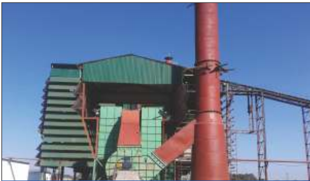
Revamped Gas Cleaning Plant
