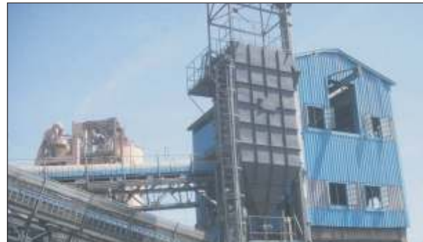
Baghouse installed on RMHS area
