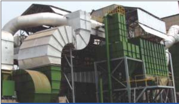
Baghouse on multifuel boiler
