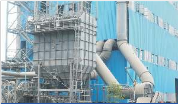
Baghouse installed on crusher house
