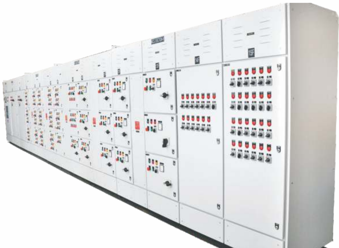
MCC panels under installation
