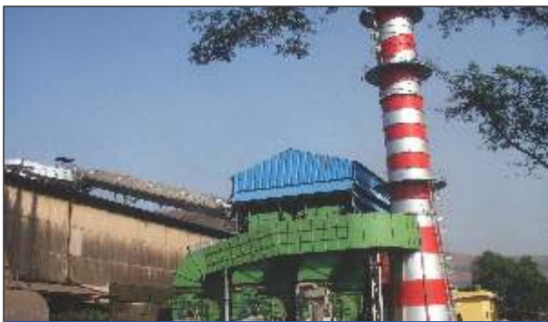
View of Secondary FES handling 600000 MCH from ID fan side
