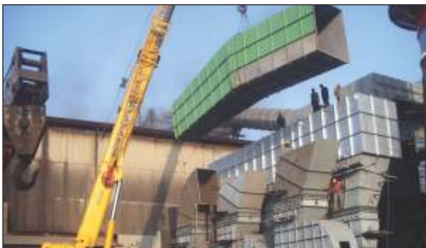
Erection of Secondary FES
