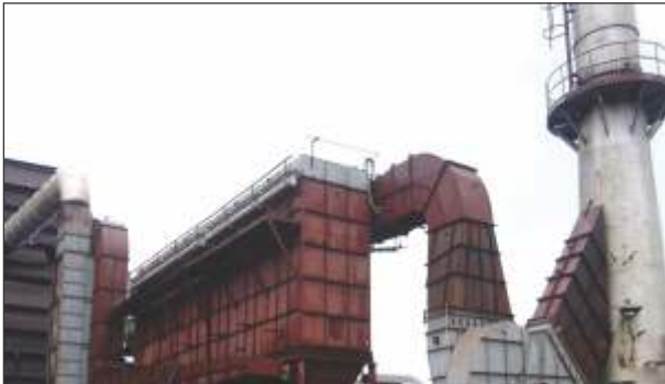
Revamped Gas Cleaning Plant on 12 MVA Furnace
