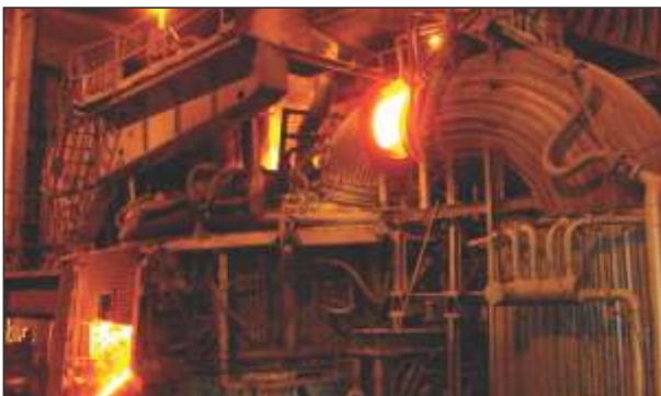
Suction at 4th hole when system in operation
