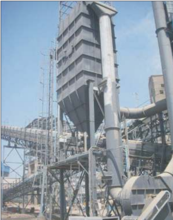
Baghouse installed on various RMHS area
