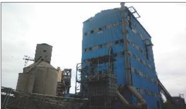
View of dust extraction system in power plant
