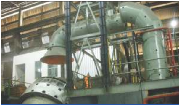
Erection of swivel hoods on AOD
