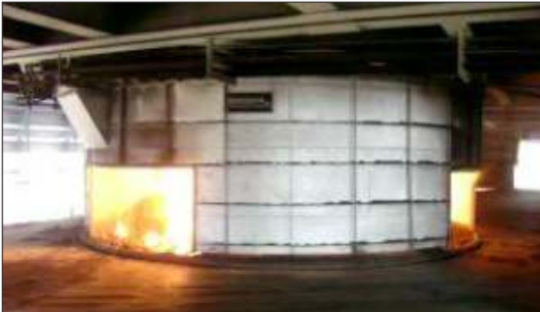
Clean work zone area near 18 MVA furnace when gas cleaning plant in operation
