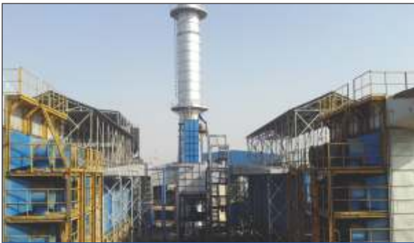
Typical view of GCP on 2 x 24 mVa furnace at OMAN
